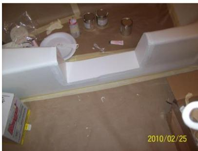
The panels have been integrated into the bathtub structure using an engineered system of metal brackets and an approved, high quality marine grade adhesive system.
